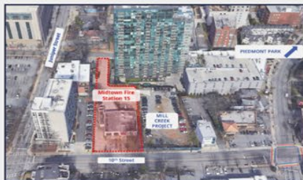
Midtown Fire Station site in Atlanta, GA, a planned high-rise development by the Atlanta Urban Development Corporation.
