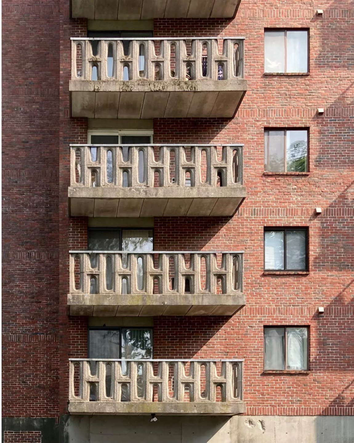
Mid-century apartments, Framingham
