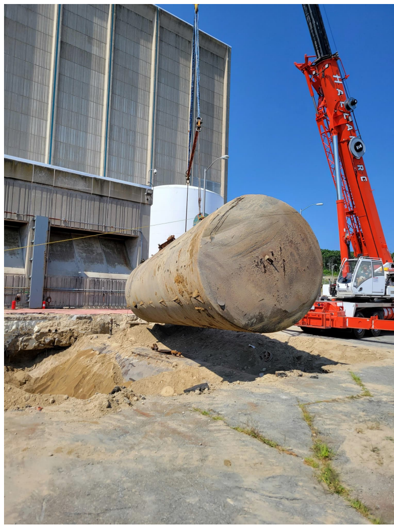
Picture showing earlier removal of Emergency Diesel Generator tank
