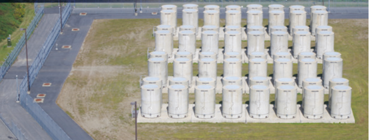
Dry cask storage at the former Maine Yankee site.
