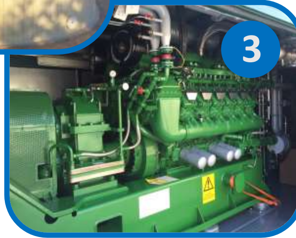
Biogas to CHP 1.2MW & 1MM BTU's
