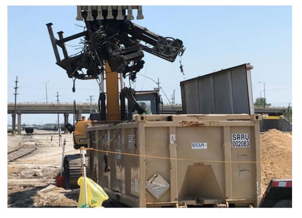
During the transloading, FRA reported and photographed large metal machinery parts, including metal shop tables, drill presses and other objects as they were removed from the car. Large pieces of wood and the remains of other combustible debris were also removed along with the Zirc Rods.
